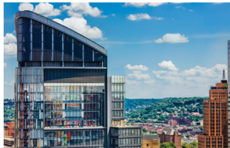
The Tower at PNC Plaza is a 33-story corporate headquarters with a design that marries pragmatism with innovation. The tower is certified LEED Platinum and features passive ventilation systems, solar chimneys, and a fully operable double-skin façade, a first in the United States.
