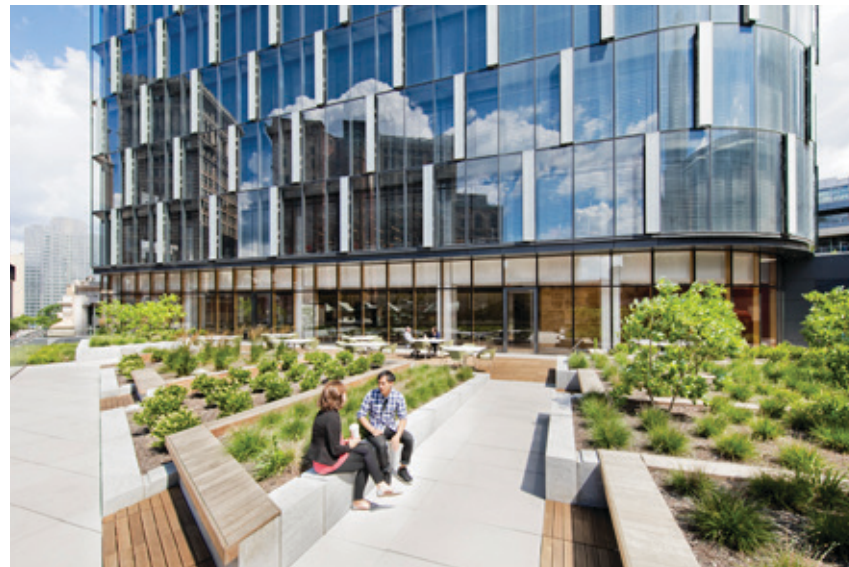
An innovative double-skin façade uses natural ventilation to breathe, which allows the tower to operate using net-zero energy for 42 percent of working hours.
