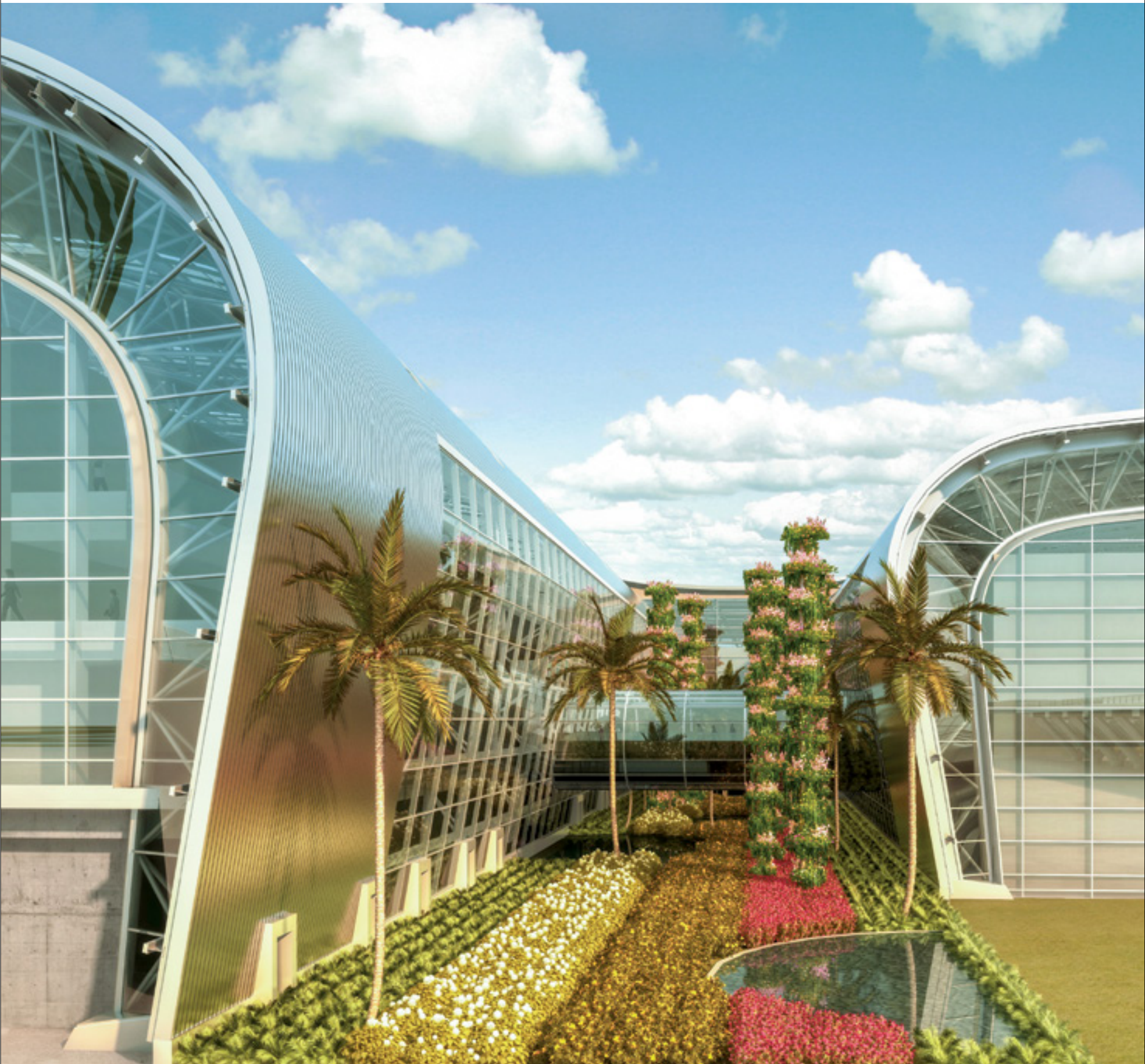
above: The expansion of India's Chennai International Airport features garden views from the new domestic and international terminals.
