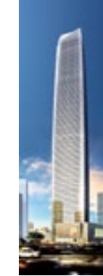
Chongqing Tianhe Tower Chongqing
