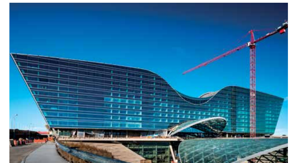
The Westin hotel at Denver International Airport topped out in May 2014. Construction of the 433,000-square-foot, 14-story hotel is slated for completion in late 2015.
