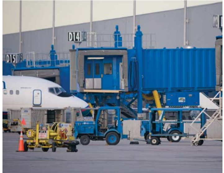
All passenger-loading bridges at Detroit Metropolitan Wayne County’s new North Terminal feature identical gangways designed without proprietary airline signage or identification.
