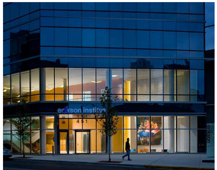
Erikson Institute’s Chicago facility is home to more than 300 students.
