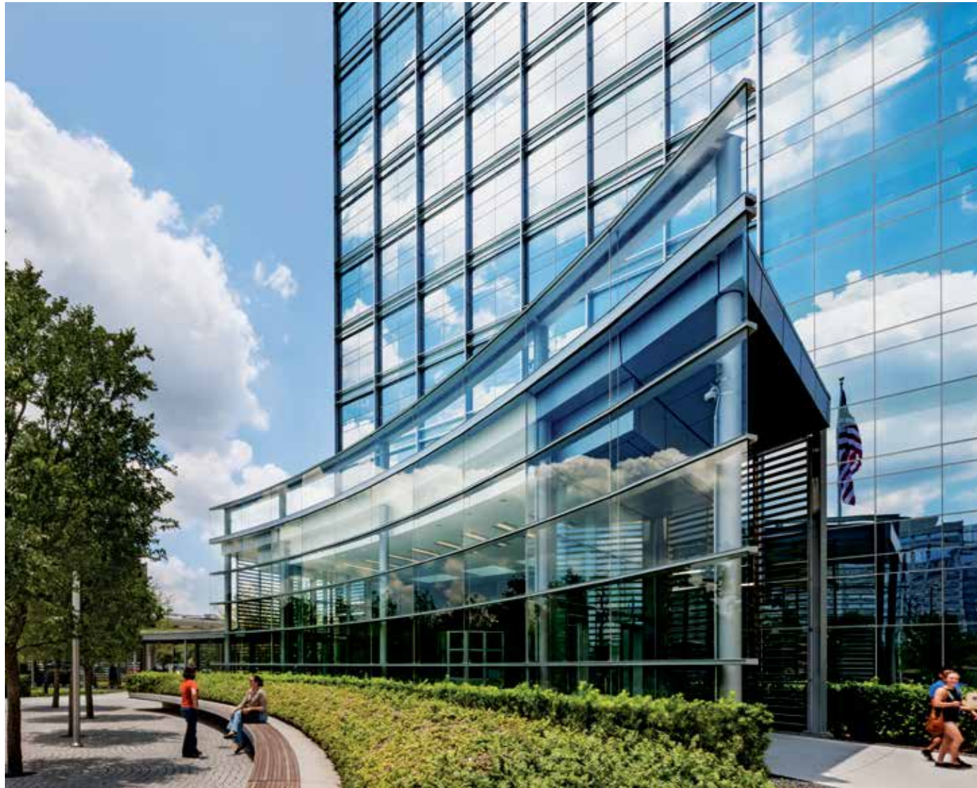
above: G.T. "Mickey" Leland Federal Building, Houston opposite: Prince Jonah Kuhio Kalaniana'ole Federal Building and U.S. Courthouse, Honolulu
