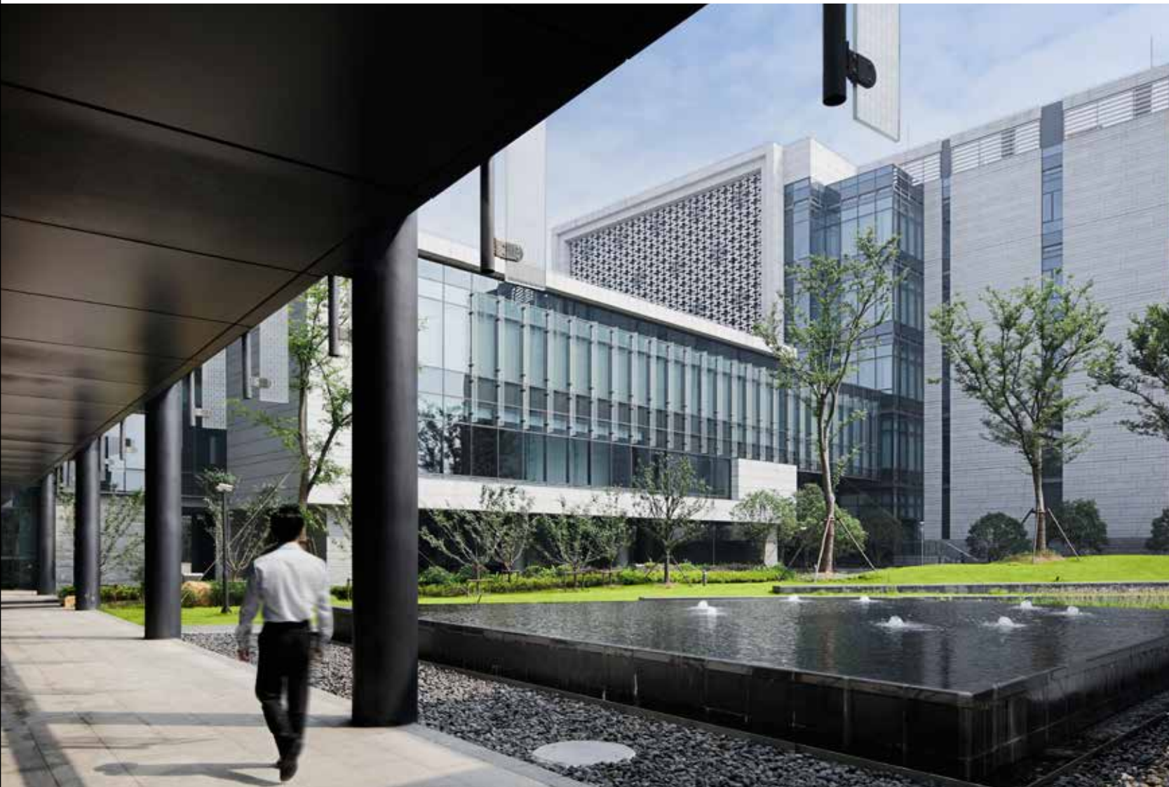
above: Confidential data and operations center, Shanghai
