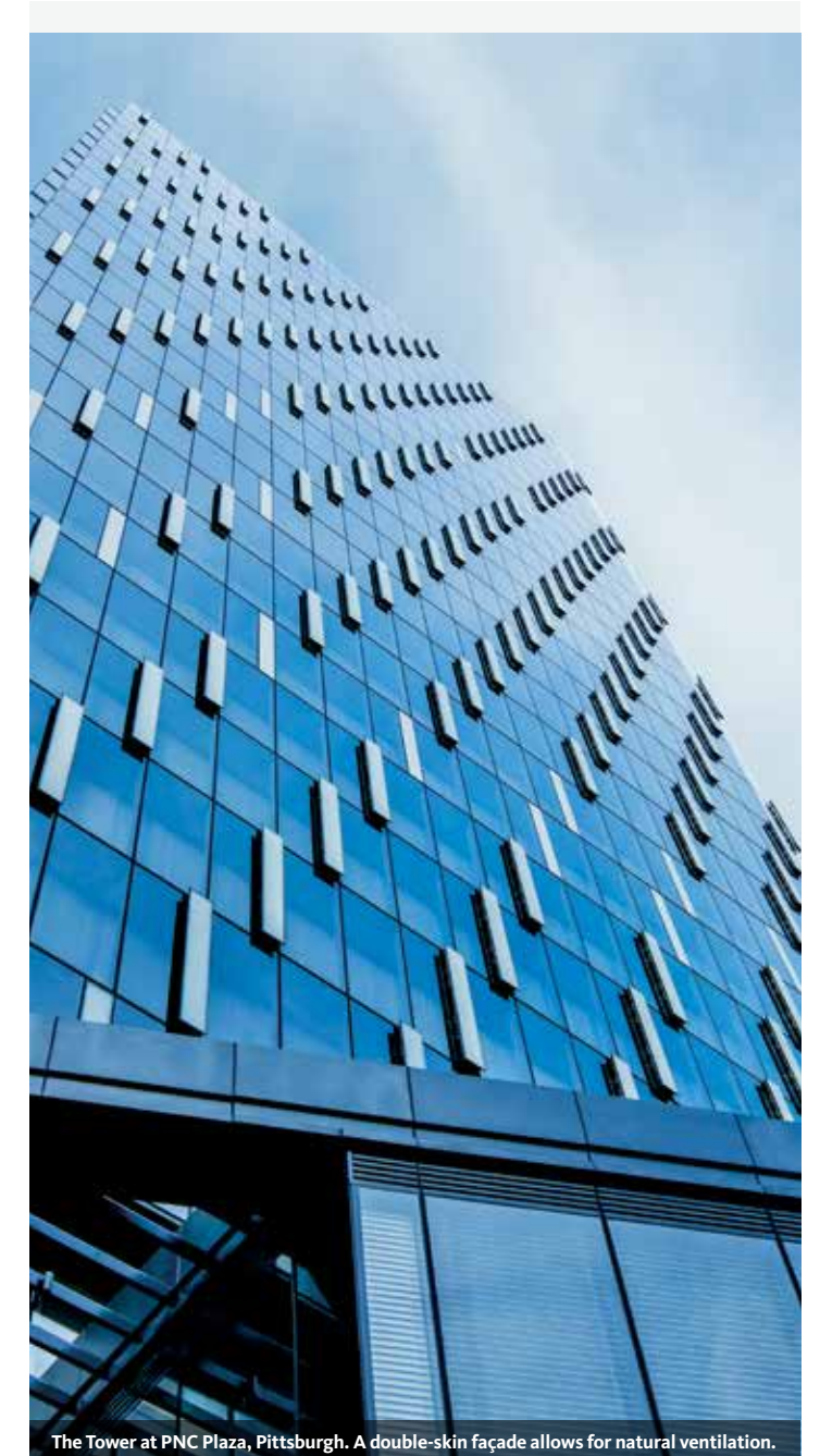
The Tower at PNC Plaza, Pittsburgh. A double-skin façade allows for natural ventilation.
